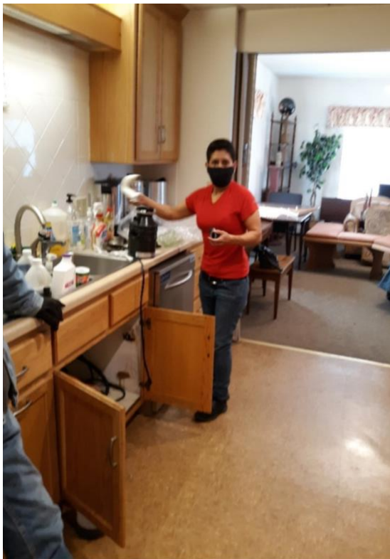
Many thanks to Soledad Beltran for installing the new Insinkerator
